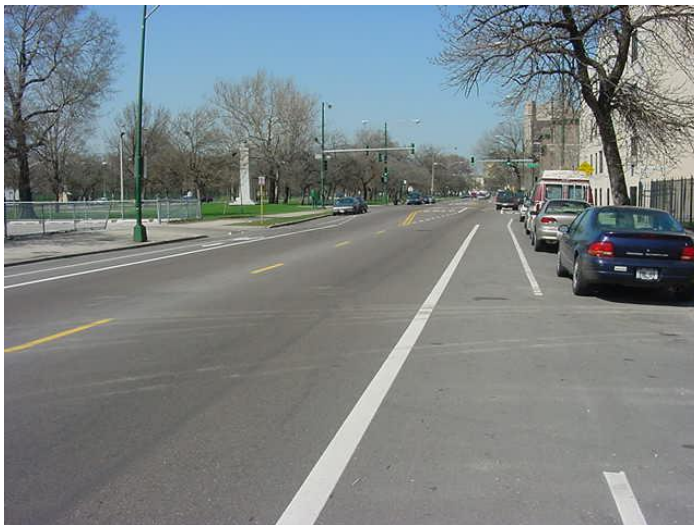
Figure A-10: Bicycle Lane with On-Street Parking
