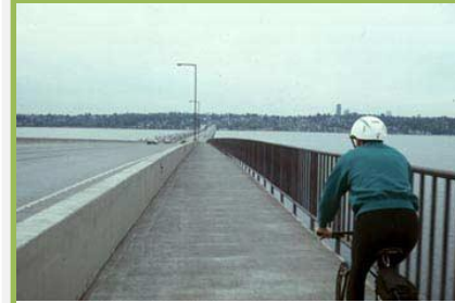
Figure A-28: Jersey barrier-protected shoulder design, Seattle
