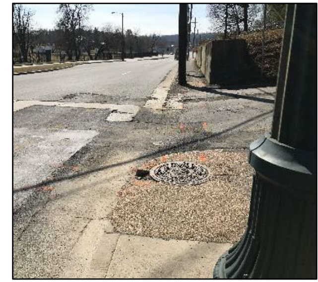
Sidewalk encroached by a utility pole on west side of the Richmond Avenue intersection
