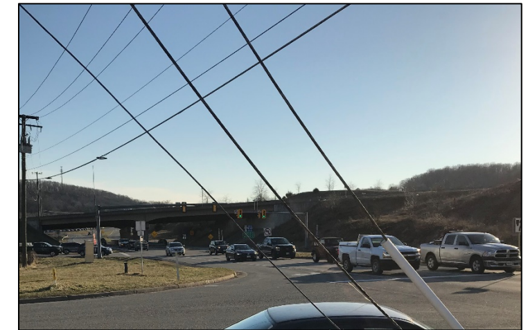
Northbound and westbound approaches of US 11 at Route 262 NB Off-Ramp intersection
