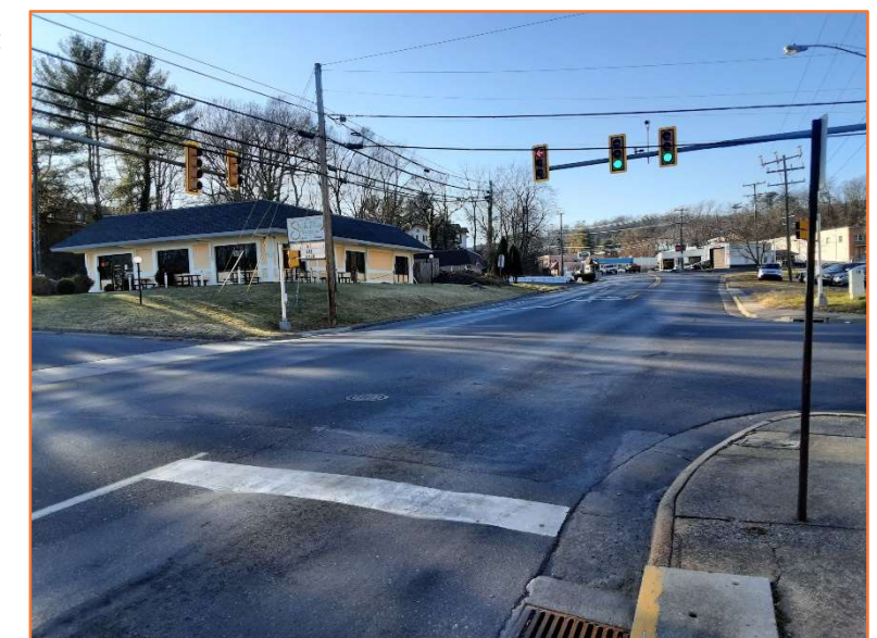
Figure 47 Site Visit Photo of W Beverley St at Grubert Ave
