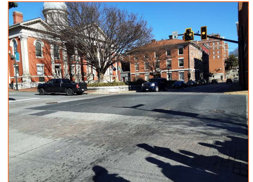
Figure 18 Site Visit Photo of W Johnson St at Augusta St
