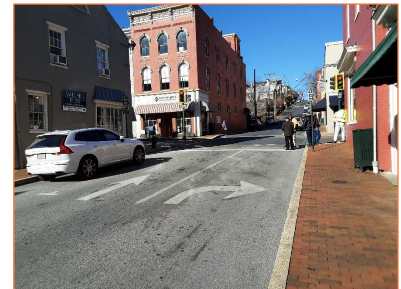
Figure 27 Site Visit Photo of W Beverley St at New St
