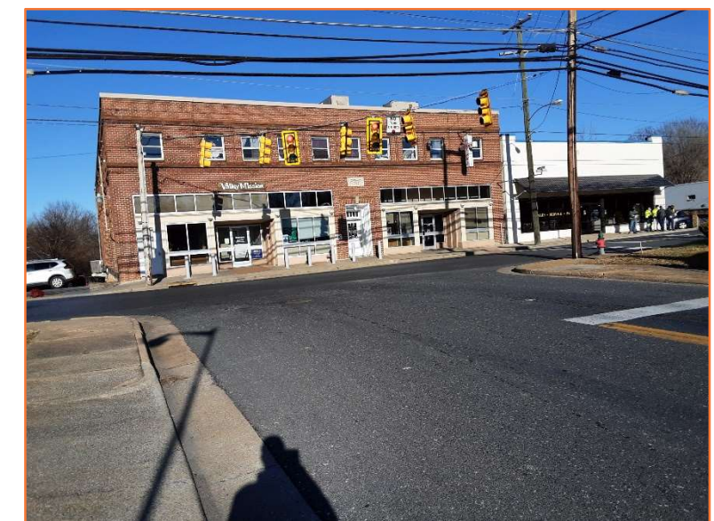
Figure 43 Site Visit Photo of W Beverley St at Hays Ave
